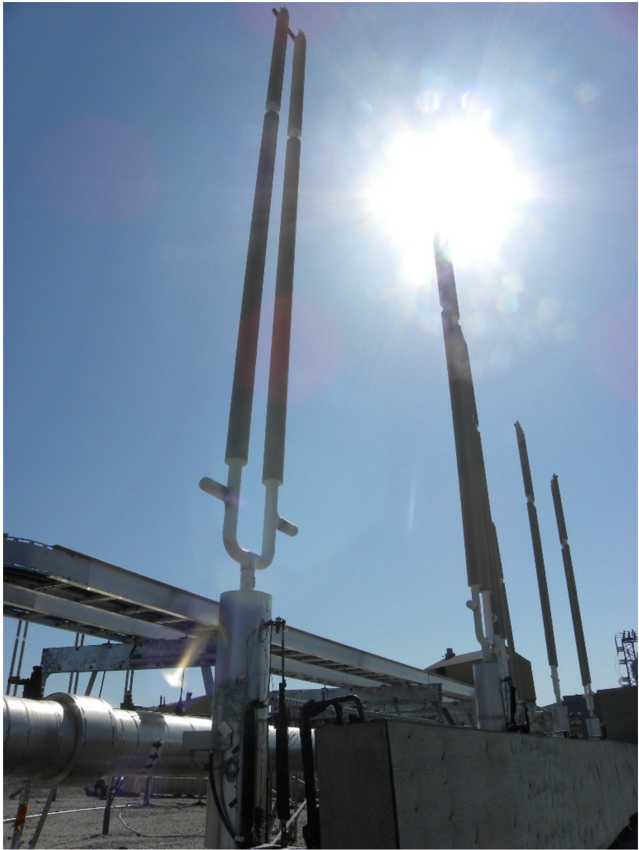
The Giant Mine thermosyphons pictured here use a passive cooling technology to freeze the arsenic
