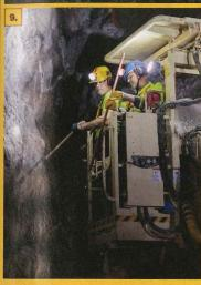
**8.** Engineers use 3-D scanners to measure the tunnels after drilling and blasting.
