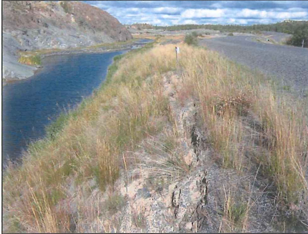
Photograph 9: Reach 4 at Baker Creek; View looking upstream at tension cracks – September 2, 2010.
