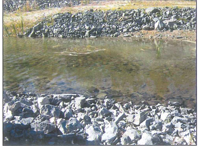
Photograph 10: Reach 4 at Baker Creek; Sideview of collapsed riffle structure – September 2, 2010.
