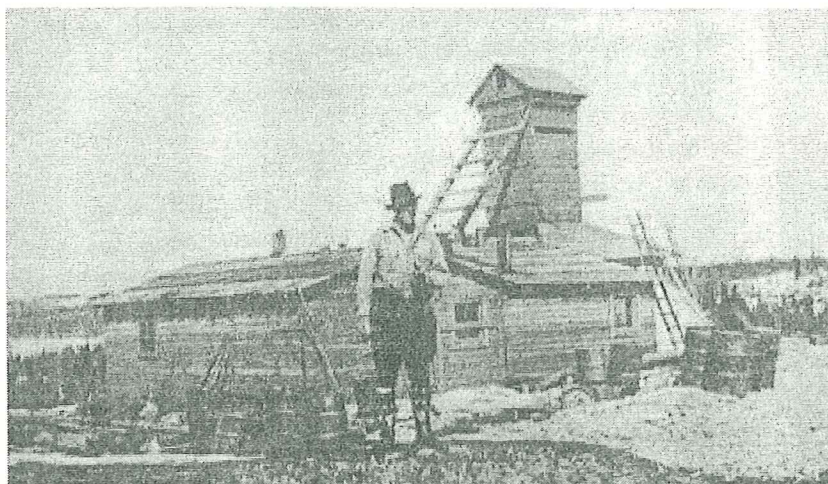
Combined powerhouse-hoist house-shaft house and headframe at Burwash, April 1936. (courtesy Susan Jackson)
