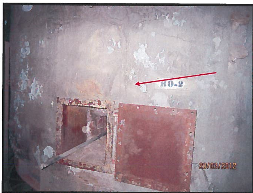
Photograph 12: Asbestos-Containing Insulation on Roaster #02 (Sample 44).
