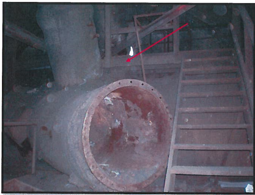
Photograph 10: Asbestos-Containing Insulation on Flue Piping located Throughout the Building (Sample 43).
