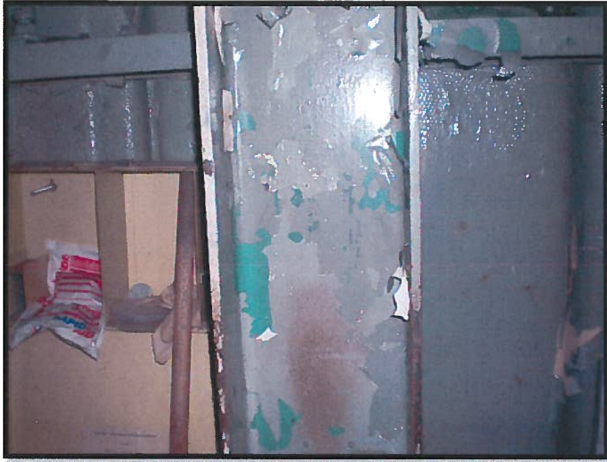
Photograph 23: Grey Paint in Control Room (Sample 17-Pb).
