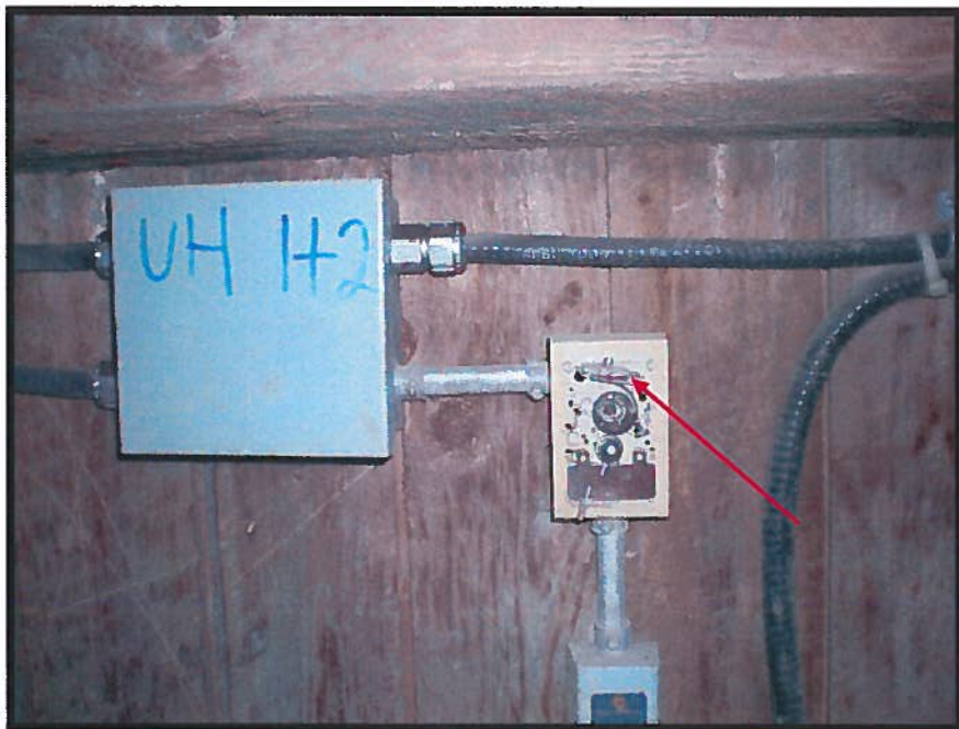
Photograph 20: Mercury-Containing Thermostat Bulbs.
