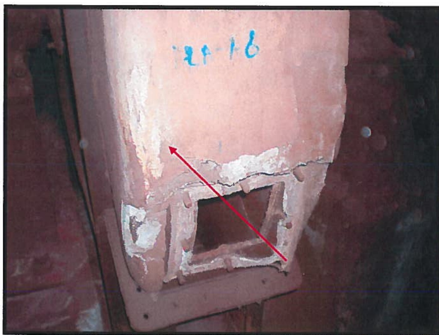
Photograph 10: Asbestos-Containing Mechanical Insulation on Equipment on Fan/Blower Unit North End (Sample 10) with suspect Asbestos-Containing Gasket Materials.
