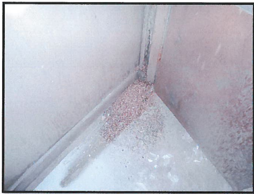
Photograph 19: Suspect Asbestos-Containing Vermiculite (not Sampled, Assumed to be contaminated with Asbestos).
