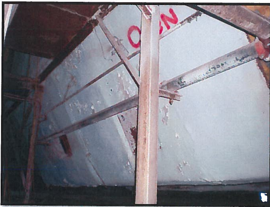
Photograph 6: Asbestos-Containing Insulation on Hoppers (Sample 1 and 2).
