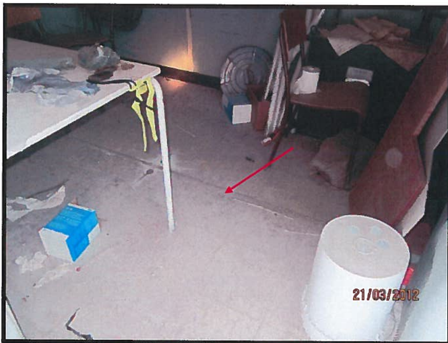
Photograph 4: Asbestos-Containing Floor Tiles in Office (Sample 54).
