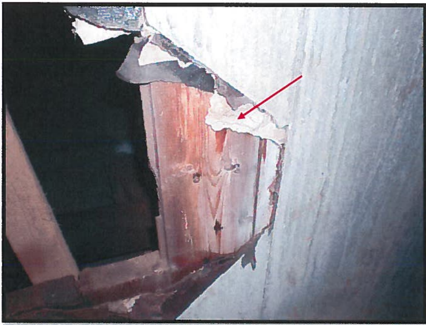
Photograph 12: Asbestos-Containing Paper Beneath Transite Wall Panels, Generator Room (Sample 36).
