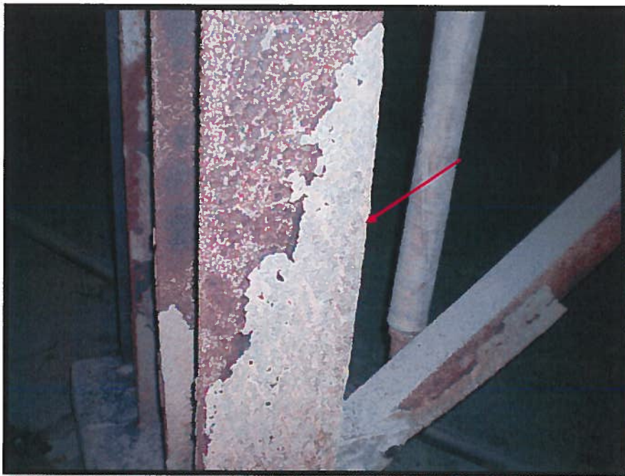
Photograph 28: Grey Paint on Structural Steel (Sample 22-Pb).
