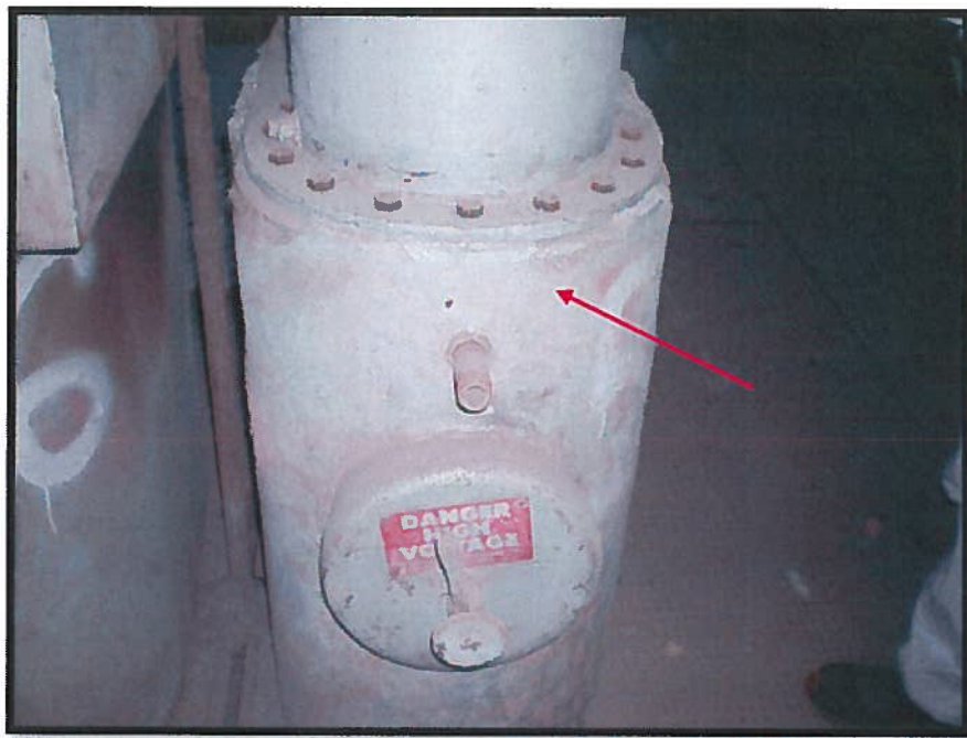
Photograph 15: Asbestos-Containing Pipe-Insulation on North Precipitator Unit Header (Sample 18).
