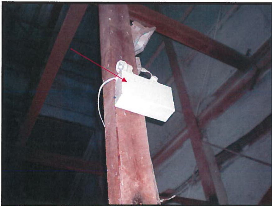
Photograph 20: Suspect Lead-Acid Batteries within Emergency Light Fixtures.
