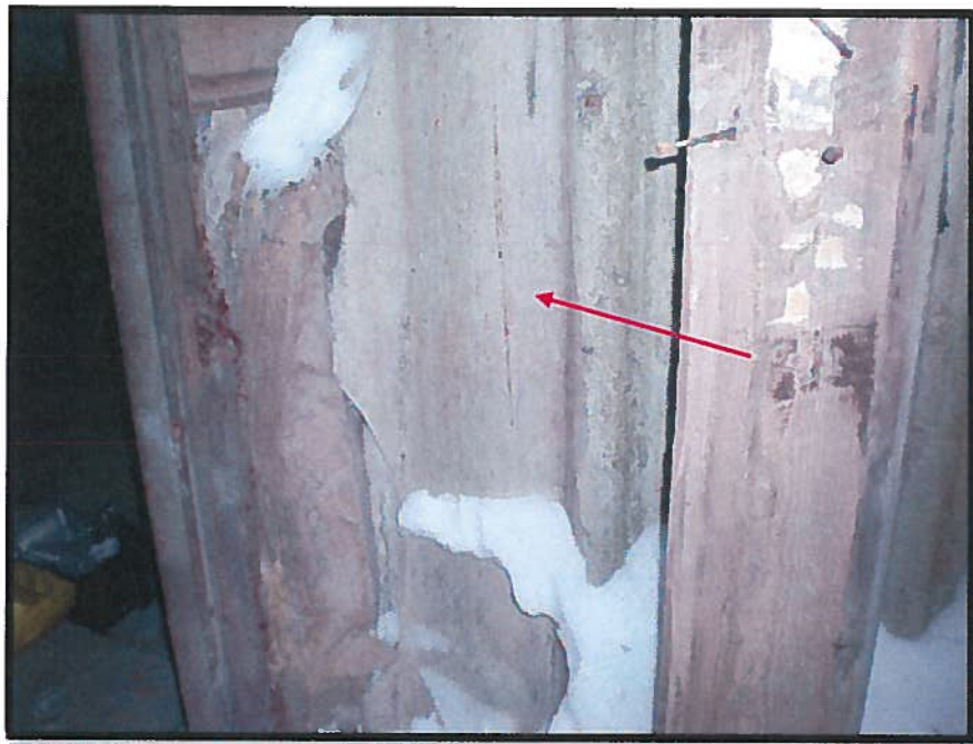
Photograph 17: Asbestos-Containing Exterior Transite Wall Panelling (Sample 20).
