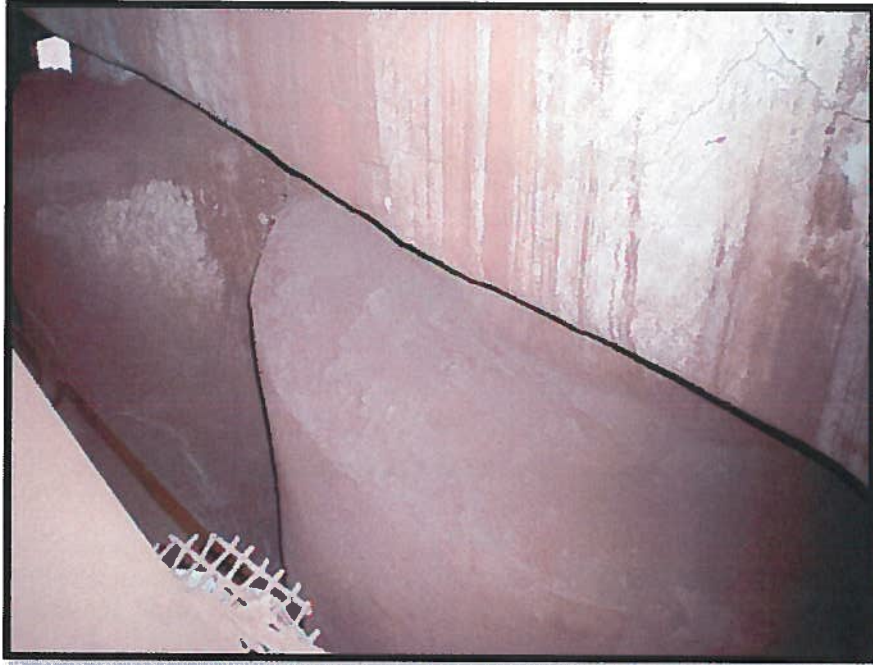
Photograph 11: Asbestos-Containing Mechanical Insulation (Sample 24).
