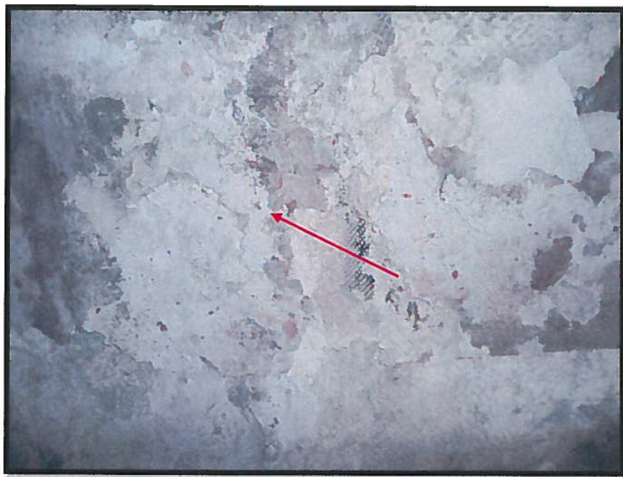
Photograph 17: Spray Applied Wall Insulation (Sample 30).
