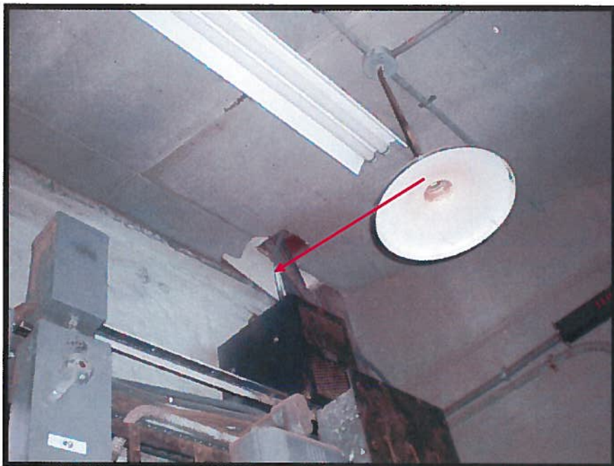
Photograph 10: Asbestos-Containing Wall Paper behind Transite Board in Electrical Room (Sample 12).
