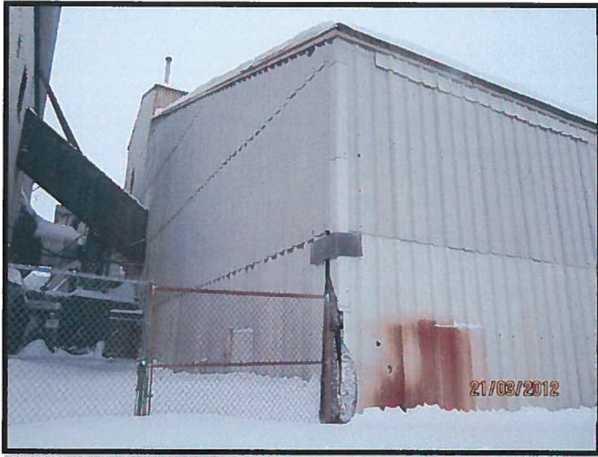
Photograph 1: Exterior of Dorrcro Roaster (North and West Walls), with typical Asbestos-Containing Exterior Panels.
