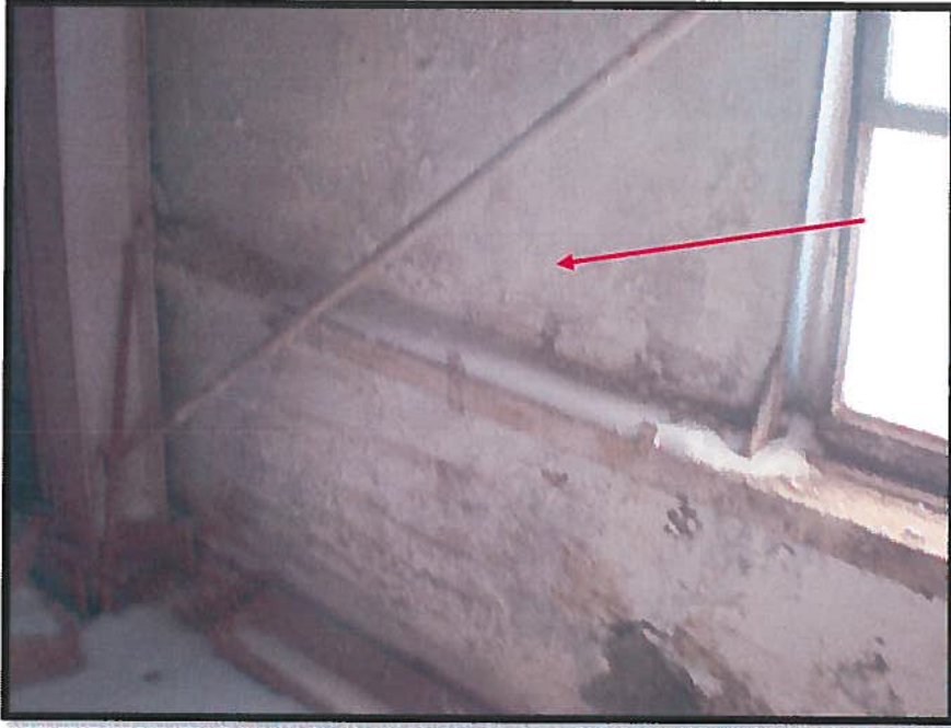
Photograph 5: Asbestos-Containing Spray-Applied Wall Insulation, South Wall (Sample 07).
