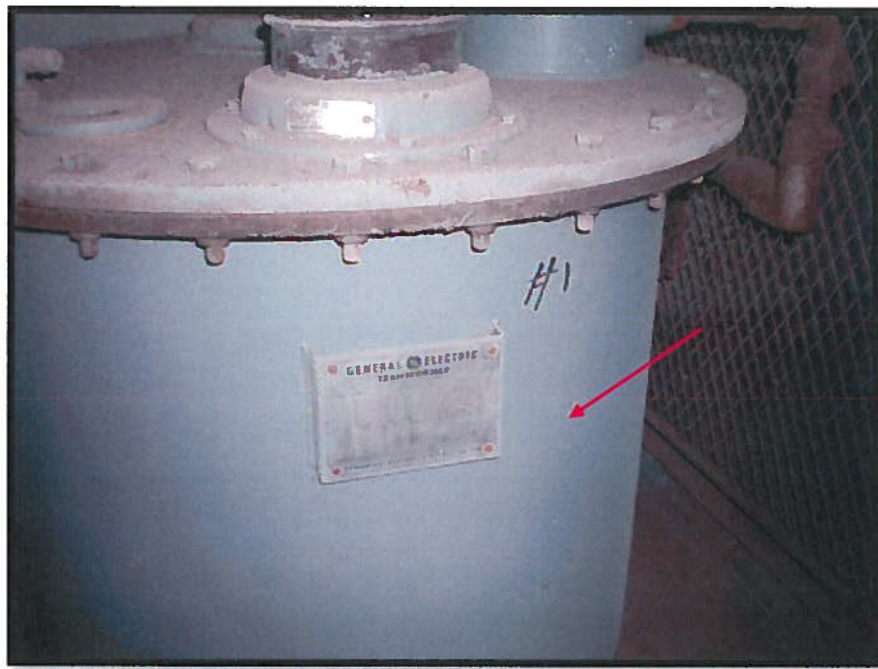
Photograph 21: Suspect PCB-Containing Oil within Transformer Unit, Upper Mezzanine Level.
