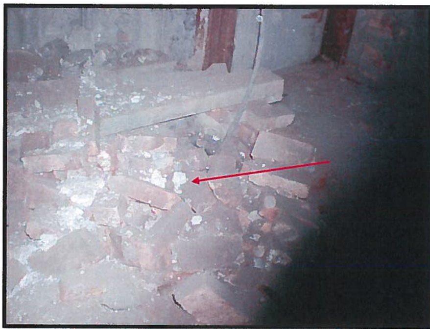
Photograph 16: Loose Refractory Bricks, (Asbestos not Detected), Adjacent Roaster #01 (Sample 51).
