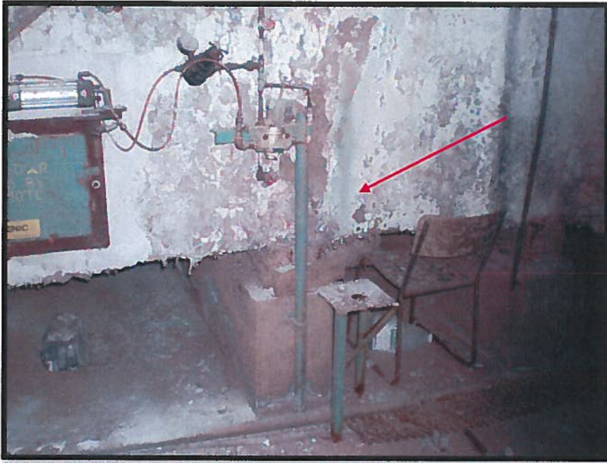
Photograph 9: Asbestos-Containing Duct Parging Insulation (Sample 11).
