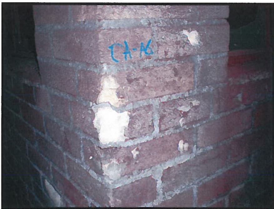
Photograph 14: Block and Mortar on Control Room (Asbestos not Detected), (Sample 27).
