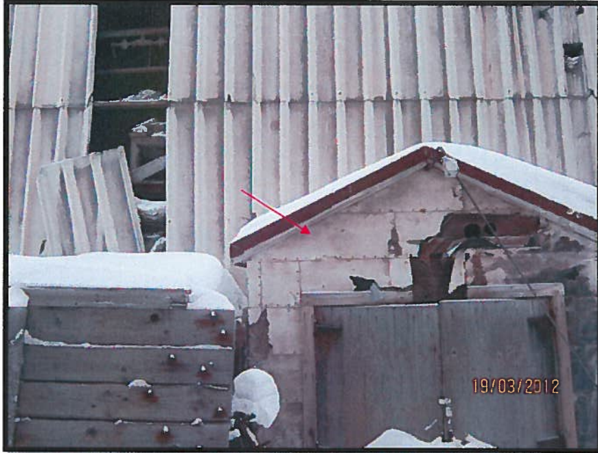
Photograph 21: Asbestos-Containing Paper Siding and Cement Panels Located on the South Wall of the Building (Visually Referenced).
