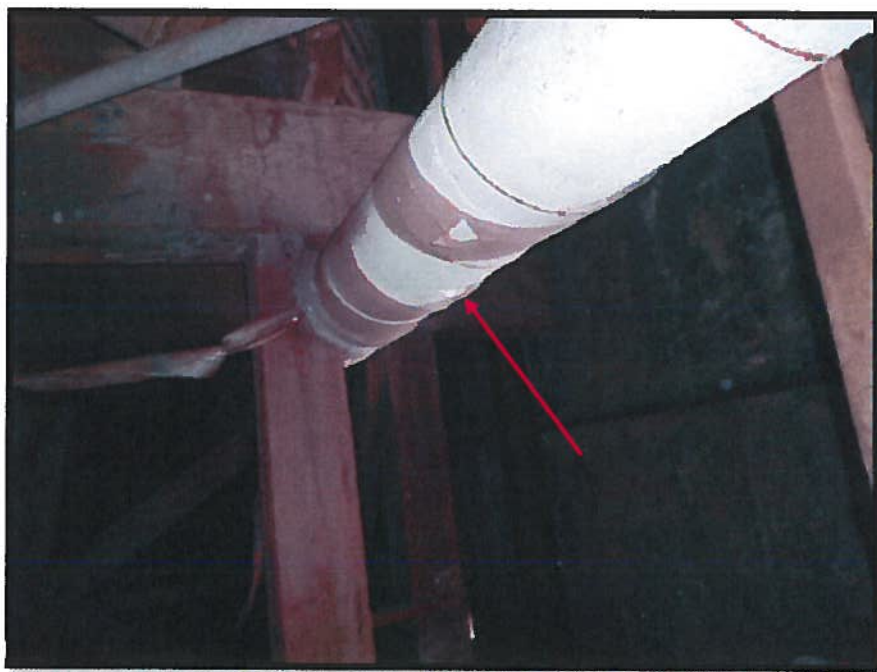
Photograph 16: Asbestos-Containing Pipe-Insulation (Sample 30).
