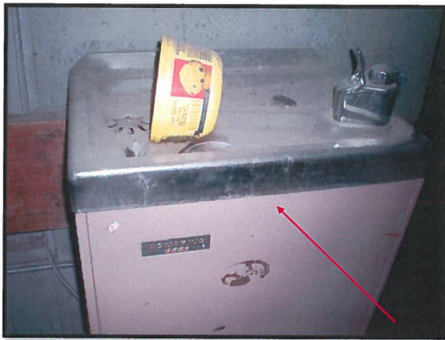
Photograph 23: Suspected ODS within Water Cooler.
