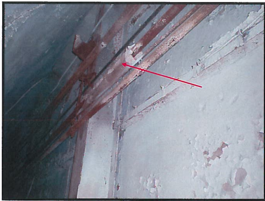
Photograph 13: Asbestos-Containing Pipe-Run Insulation Adjacent to Stairwell (Sample 16).
