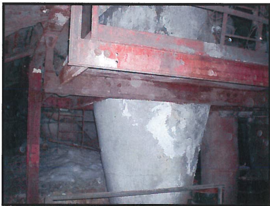
Photograph 20: Typical Mechanical Insulation on Flue Network Cyclones (Visually Referenced, Sample 43).
