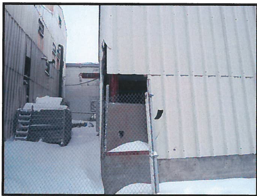
Photograph 8: Asbestos-Containing Exterior Wall Panels (Sample 21).
