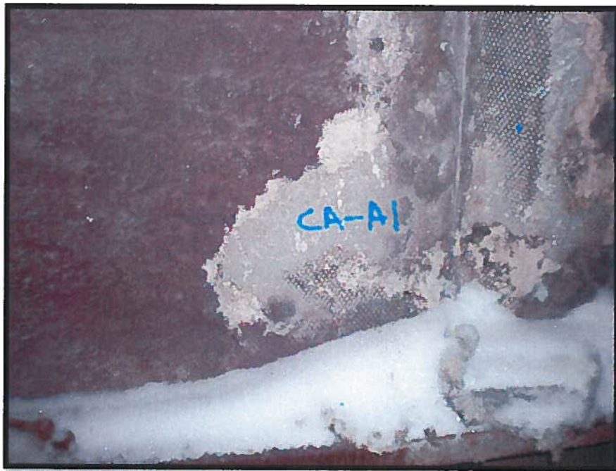
Photograph 12: Spray Applied Asbestos-Containing Wall Insulation (Sample 25).
