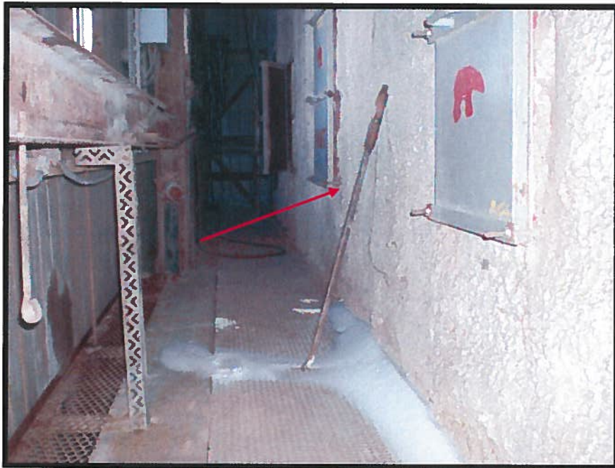
Photograph 8: Asbestos-Containing Insulation on Bag Compartment Walls (Samples 3 and 4).
