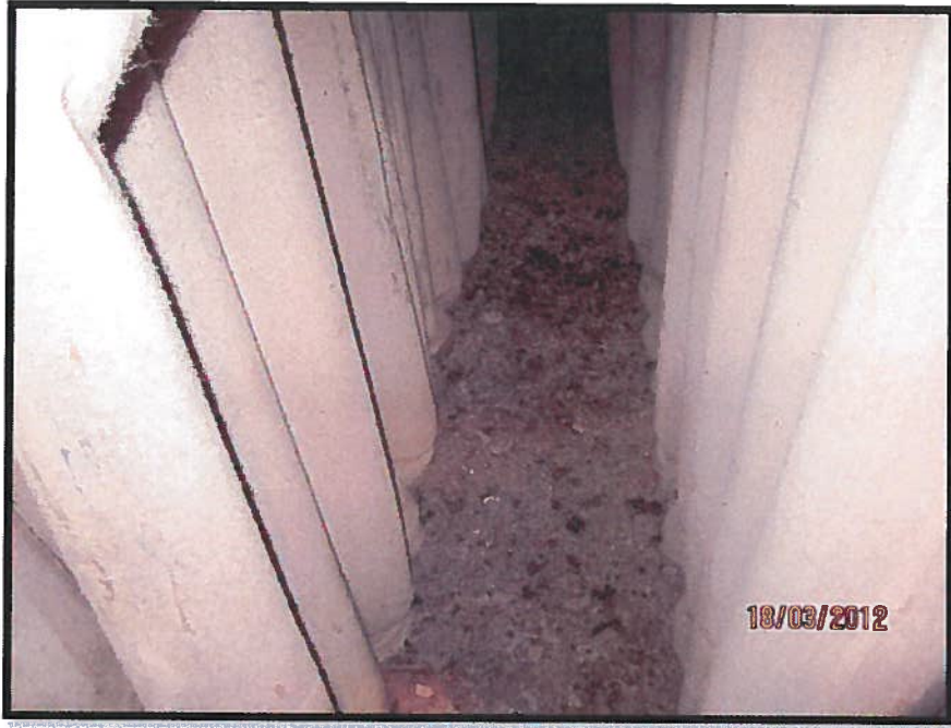
Photograph 5: Inside Baghouse Compartments (Suspect Arsenic Contaminated Debris and Filter Bags).
