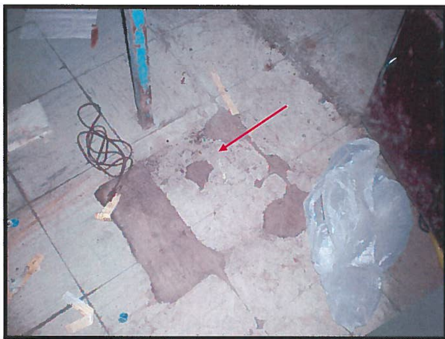
Photograph 12: Asbestos-Containing Floor Tiles within Control Room/Office (Sample 15).
