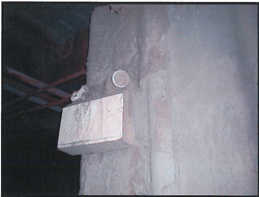
Photograph 30: Emergency Light Fixture with Lead-Acid Batteries.
