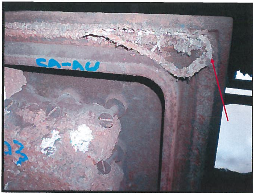
Photograph 15: Asbestos-Containing Gasket on Furnace Door (Sample 28).
