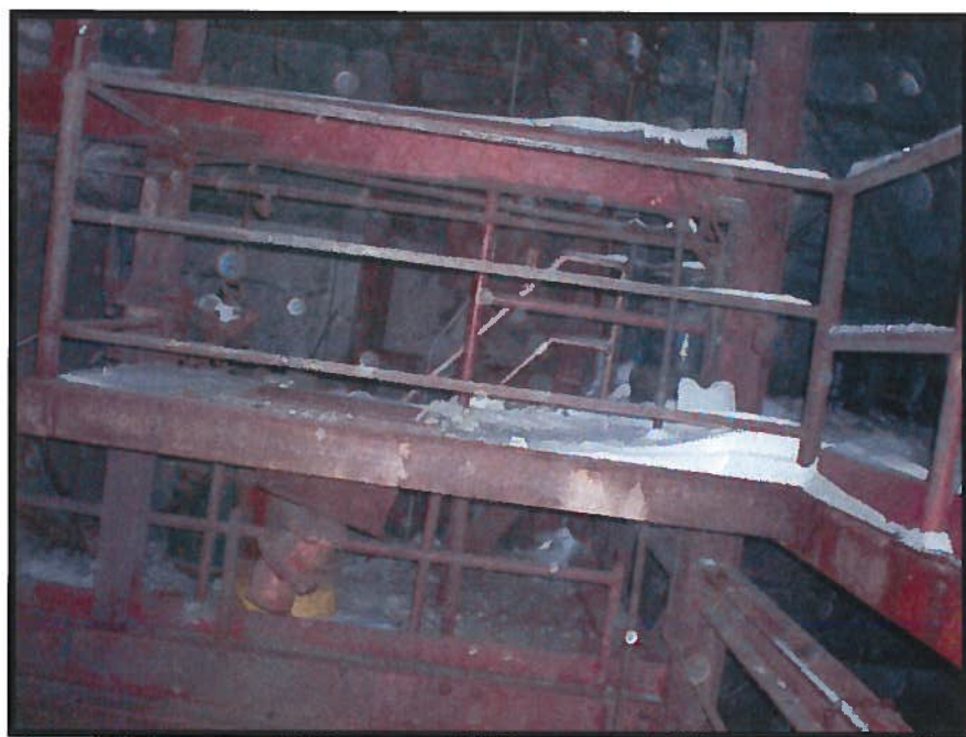
Photograph 26: Red Paint on Structural Steel (Sample 20-Pb).
