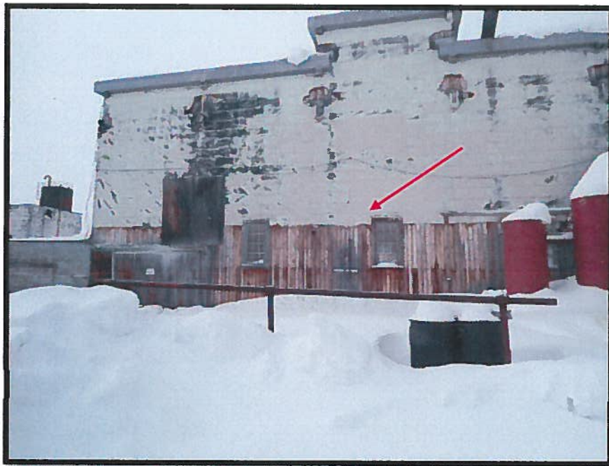
Photograph 15: Asbestos-Containing Exterior Siding Paper (Sample 39).
