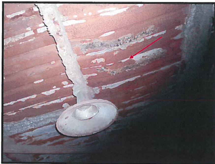
Photograph 7: Delaminating Ceiling Insulation Materials, Non-Asbestos (Sample 31).
