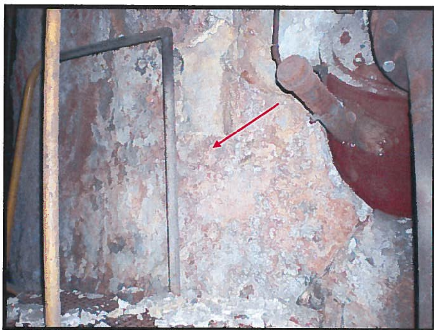
Photograph 14: Asbestos-Containing Insulation Roaster #01 (Sample 47).
