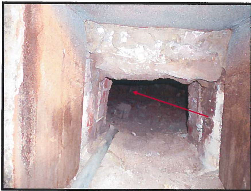
Photograph 18: Suspect Asbestos-Containing Refractory Bricks and Linings (not accessible).
