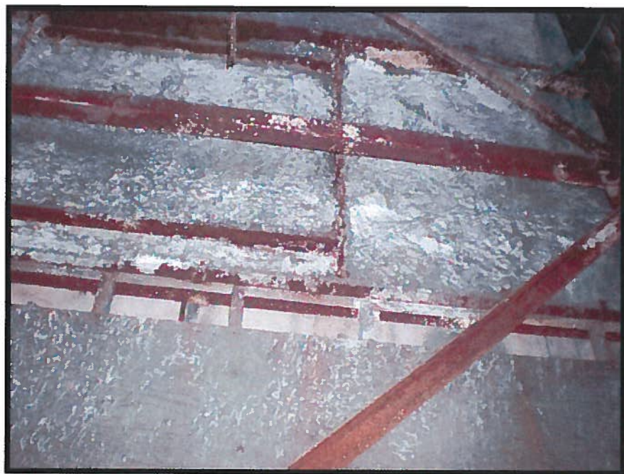
Photograph 10: Typical Asbestos-Containing Spray-Applied Wall Insulation.
