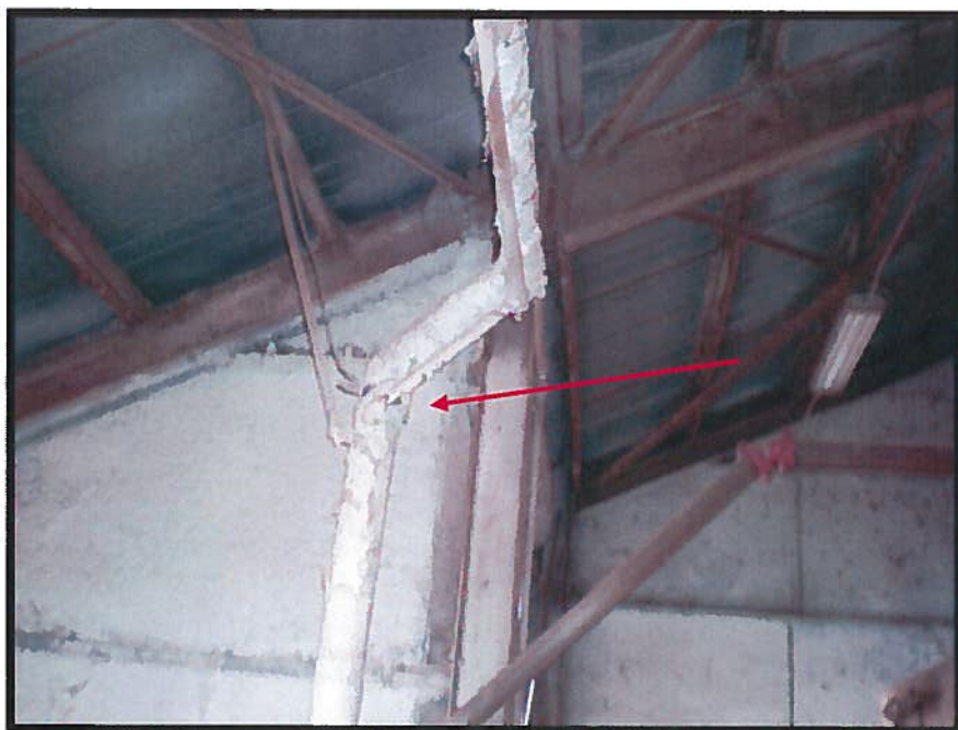
Photograph 14: Asbestos-Containing 4" Pipe-Run Insulation (Sample 17).
