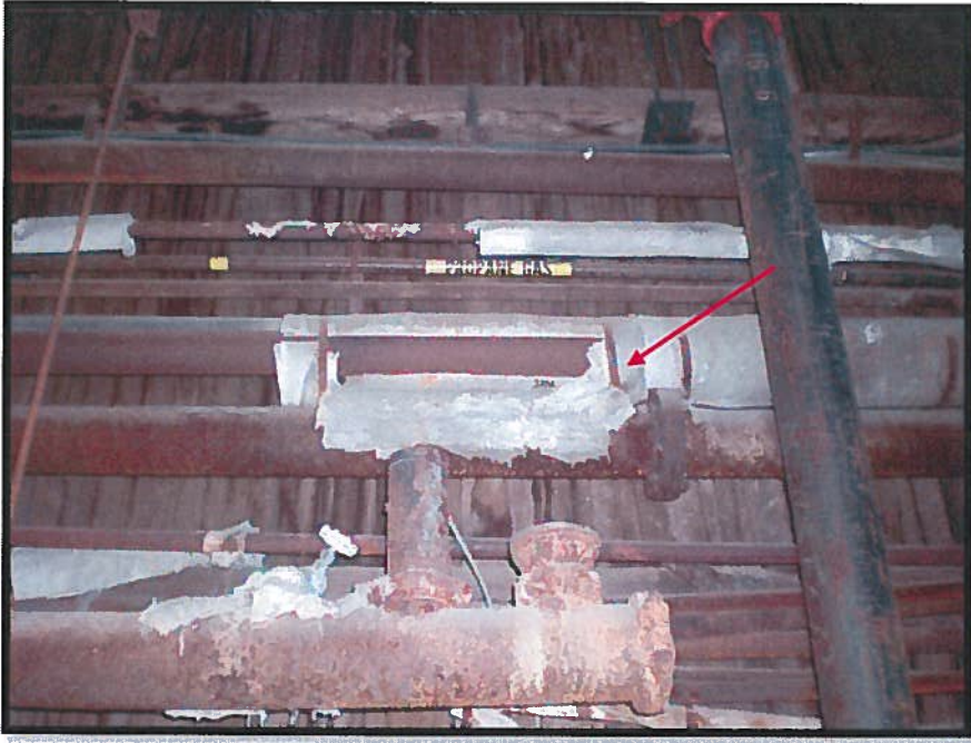
Photograph 9: Asbestos-Containing Pipe-Run Insulation along Perimeter Walls (Sample 31).
