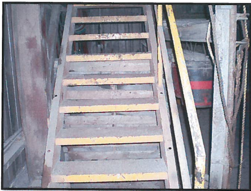
Photograph 9: Yellow over Green Paint on Stairway (Sample 01-Pb).
