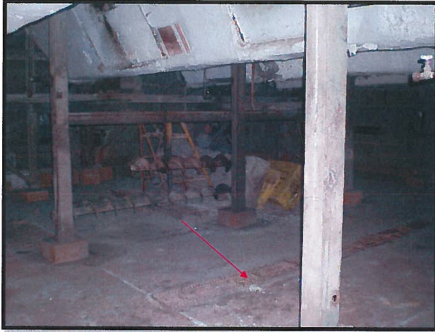
Photograph 7: Asbestos-Containing Insulation on Hoppers (Samples 1 and 2) with Minor Amounts of Insulation Debris on the Ground.
