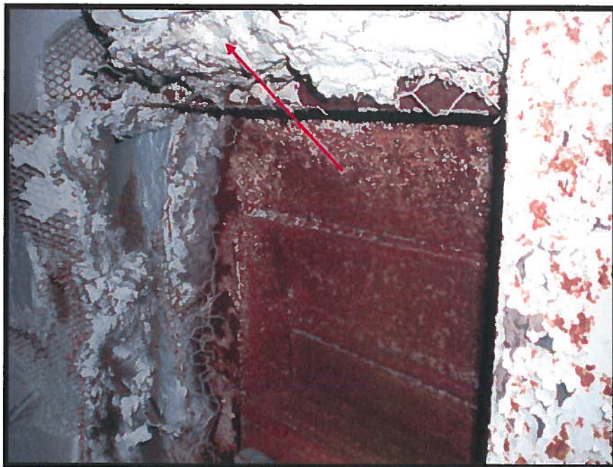
Photograph 8: Asbestos-Containing Precipitator Vessel Insulation, South Vessel (Sample 10).
