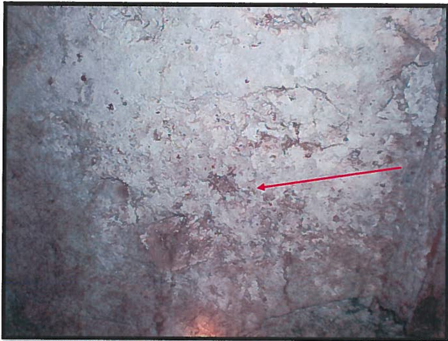
Photograph 6: Asbestos-Containing Spray-Applied Wall Insulation, West Wall (Sample 08).
