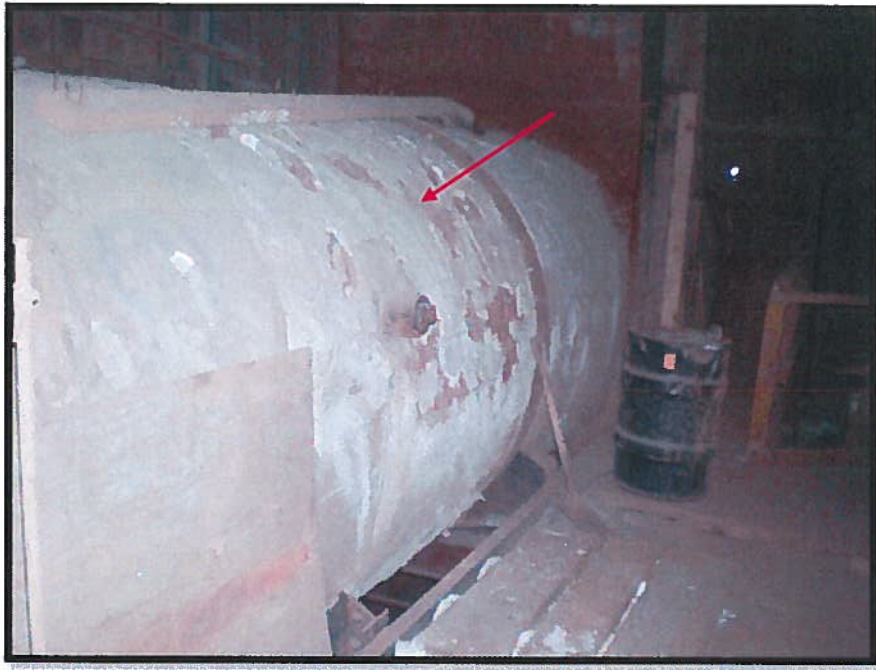
Photograph 11: Asbestos-Containing Flue-Pipe Insulation (Sample 34).
