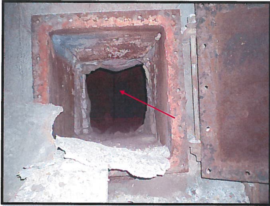
Photograph 17: Suspect Asbestos-Containing Refractory Bricks and Linings (not accessible).
