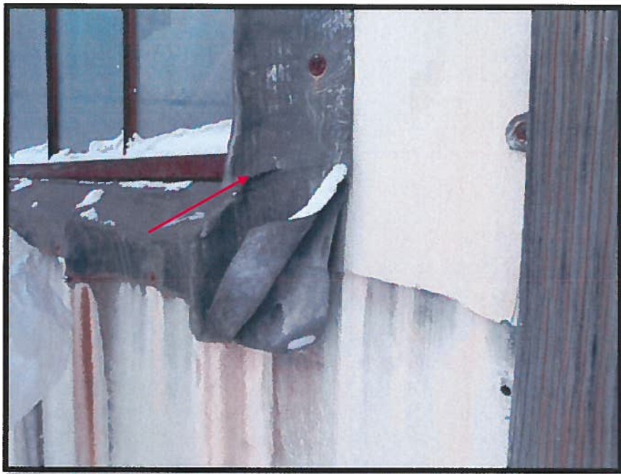
Photograph 3: Lead Sheeting around Exterior Window Frames.
