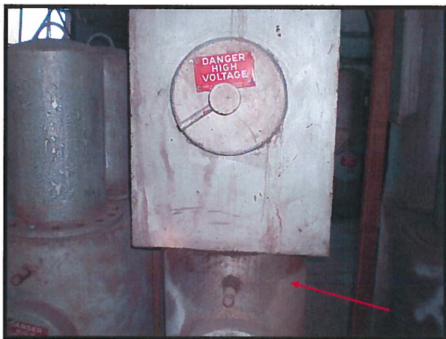
Photograph 16: Asbestos-Containing Pipe-Insulation on South Precipitator Unit Header (Sample 19).
