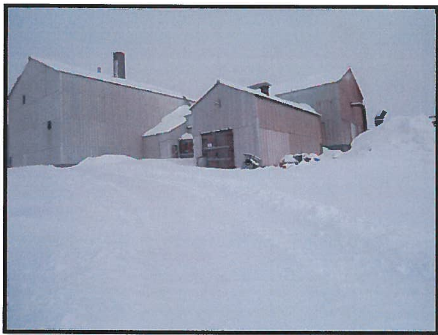
Photograph 1: Calcine Building (Three Visible Phases/Buildings). Asbestos-Containing Exterior Siding and Roofing is Visible.
