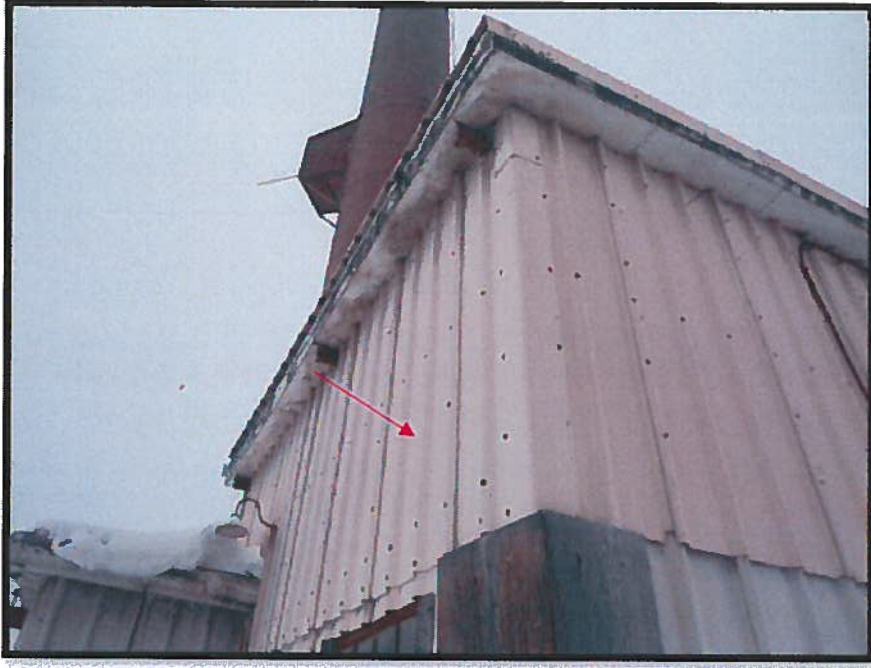
Photograph 1: Asbestos-Containing Cement Board Panels On Building Exterior (Visually Referenced).
