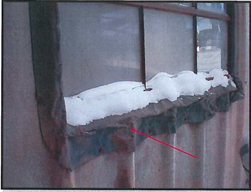
Photograph 19: Lead Sheeting around Exterior Windows.
