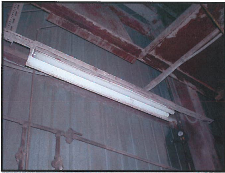
Photograph 15: Typical Fluorescent Light Fixture with Mercury-Vapour Tubes and Suspect PCB-Containing Ballasts.
