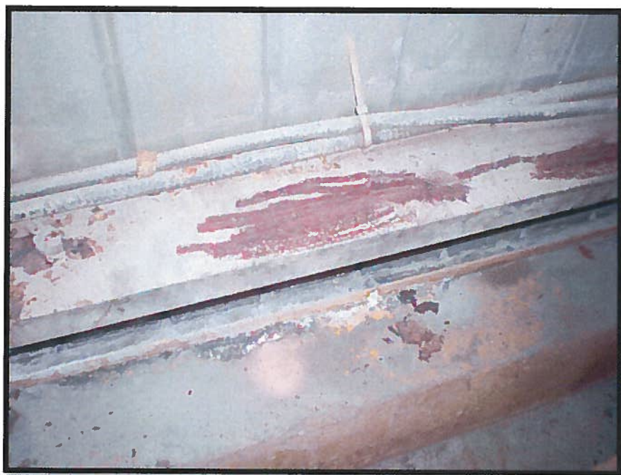
Photograph 10: Silver over Red Paint on Structural Steel and Yellow Paint on Concrete (Samples 02-Pb and 03-Pb).
