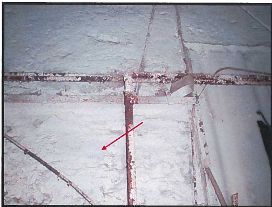
Photograph 4: Asbestos-Containing Spray-Applied Wall Insulation, East Wall (Sample 06).
