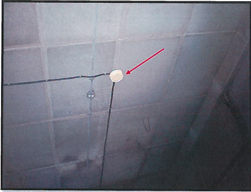
Photograph 21: Suspect Radioactive Components within Ceiling Smoke Detector.
