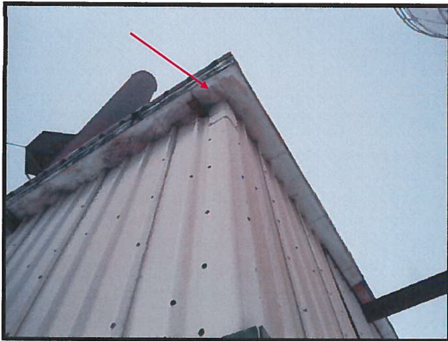
Photograph 2: Asbestos-Containing Exterior Siding Paper (Visually Referenced).
