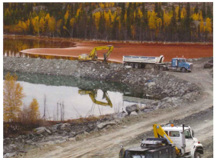
Working on the split dyke between the settling and polishing ponds at Giant Mine
