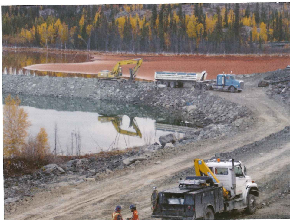
Raising the filter dyke between the settling and finishing ponds
