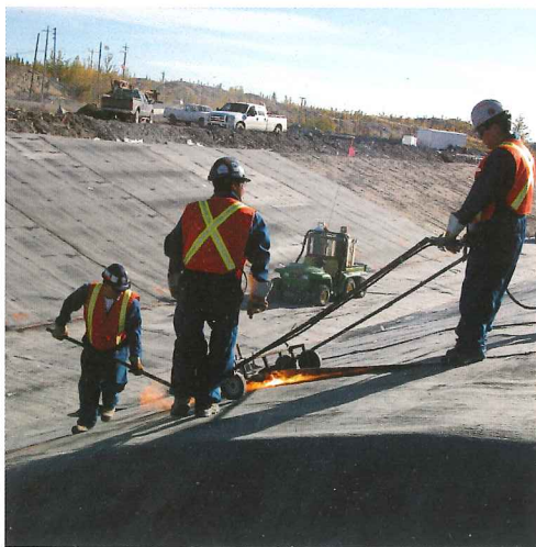
Placing bitumen liner in the new creek bed
