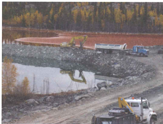
Working on the split dyke between the settling and polishing ponds at Giant Mine.
