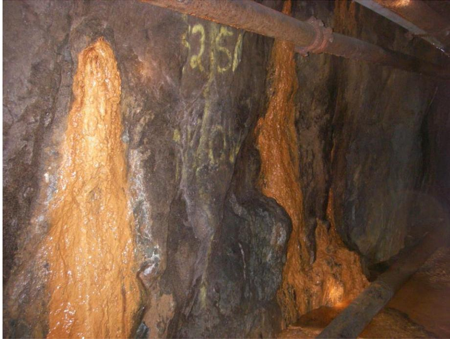
**Figure 1: Biofilms formed from arsenite-bearing groundwater seeps in underground workings at Giant Mine (Photo courtesy of S. Simpson, Lorax Consulting)**
