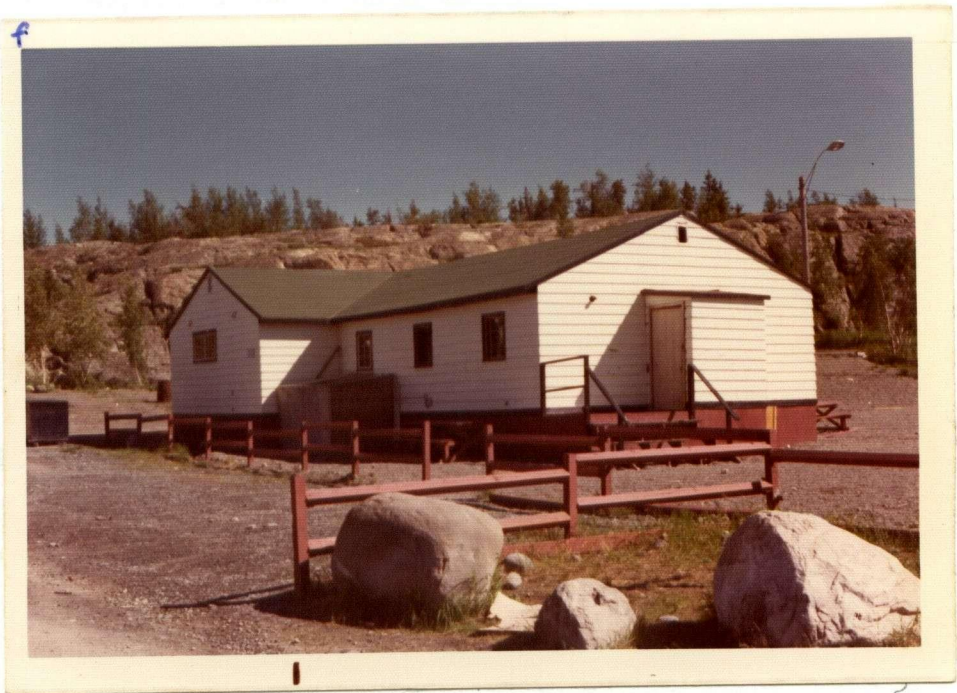
Photograph 4.6 : The Latham Island Community Centre.
