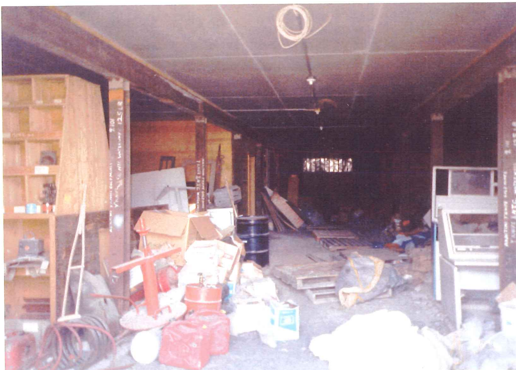
Lower Level Showing Storage Items and Asbestos Type 1 on Ceiling
