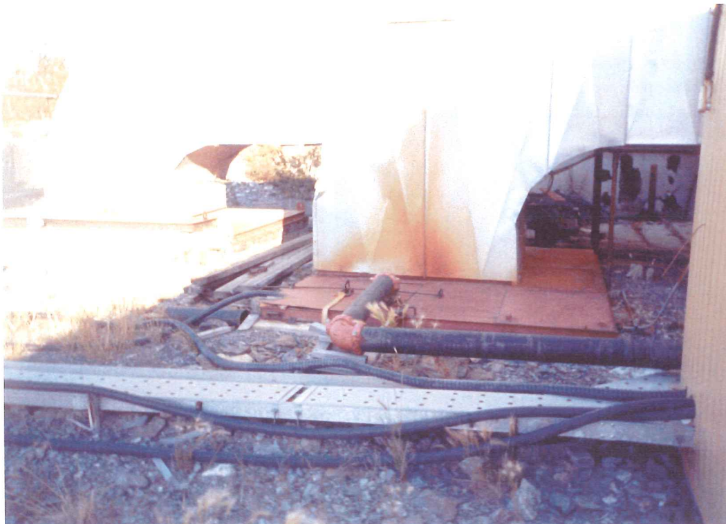
Fan and Housing Ventilation Showing Shaft Locations
