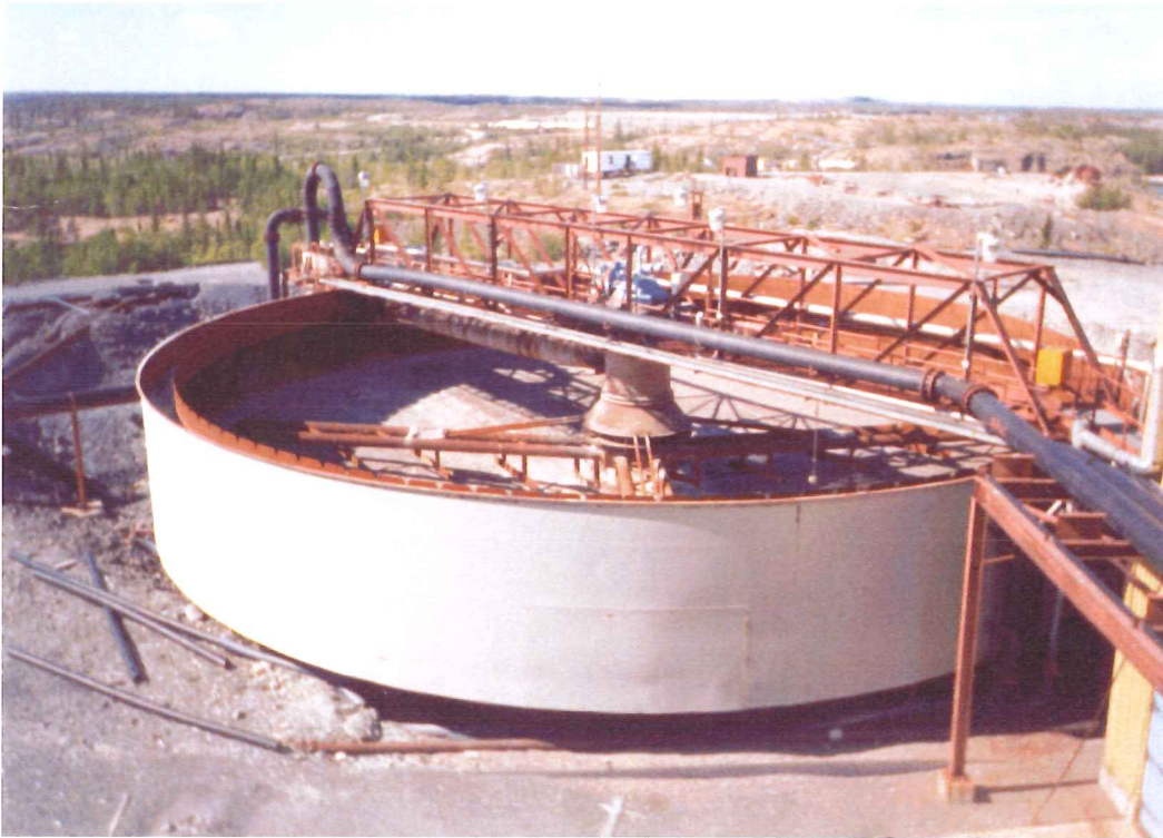
Typical Thickener Steel Construction
