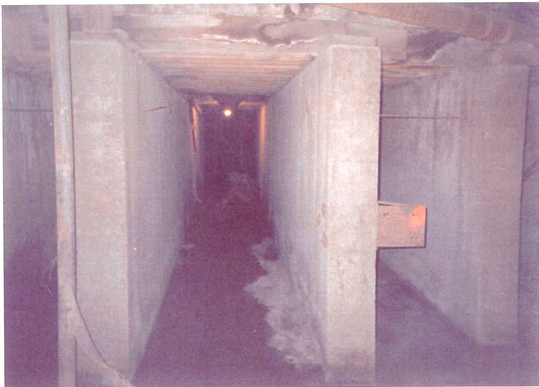
Typical Concrete Supports for Tanks
