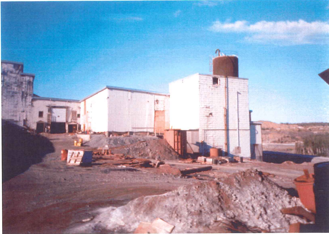
Mill Looking Southwest Showing Exterior Asbestos Siding Type 1 and Lime Silo
