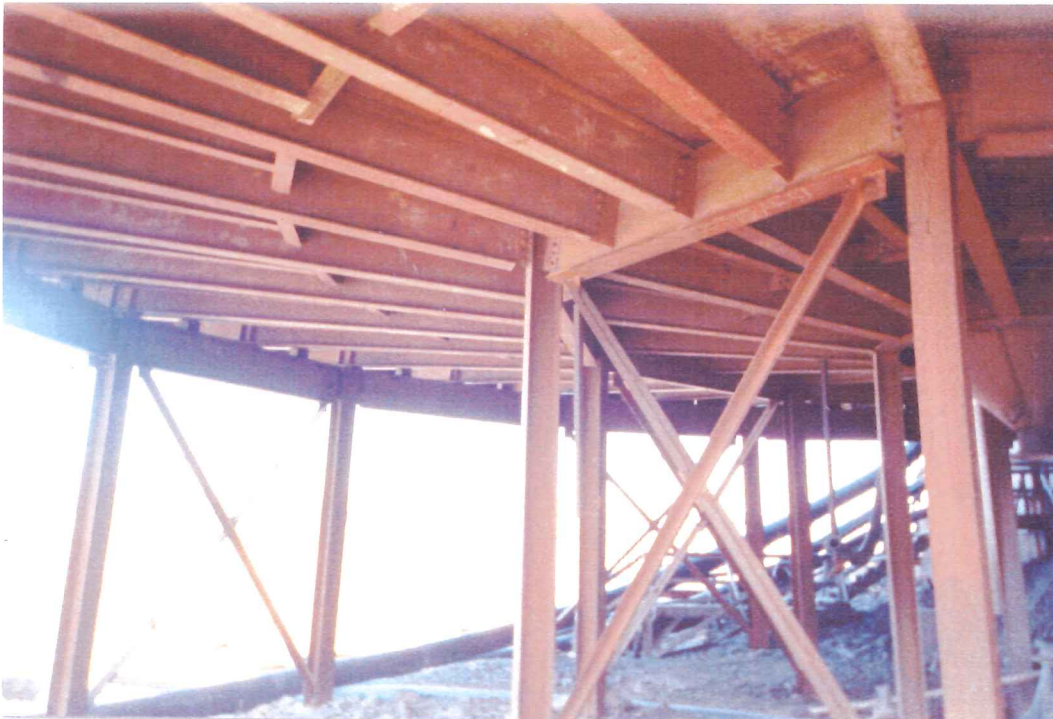
Typical Thickener Steel Construction
