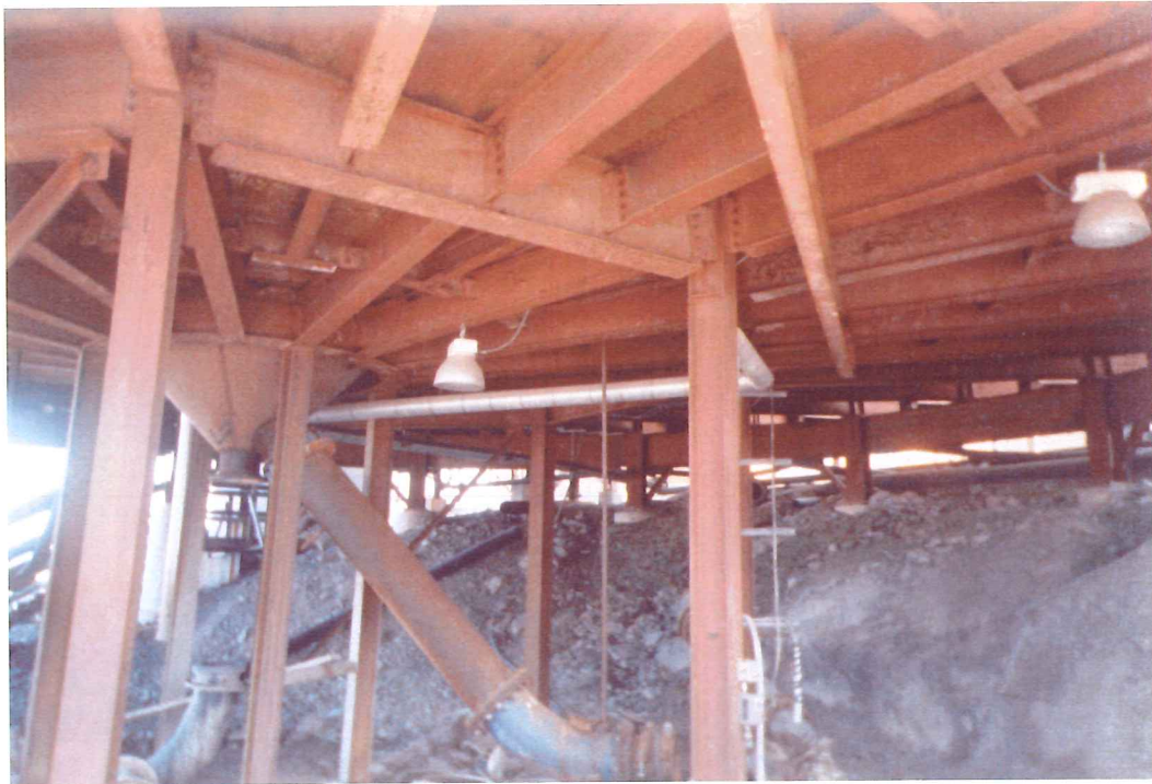
Typical Thickener Support Steel
