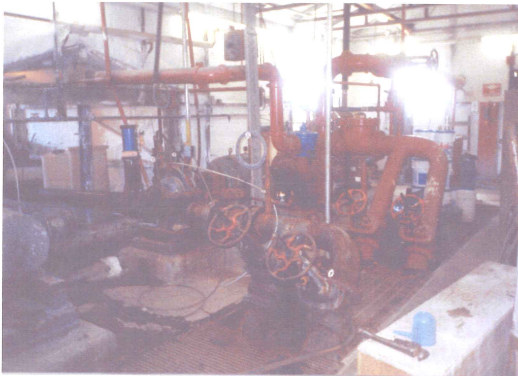
Typical Interior Piping - Asbestos Type 2 on Walls
