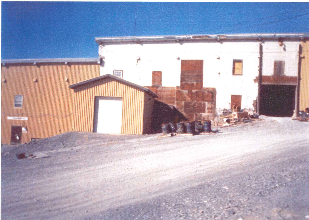
Mill Looking North Note Steel Siding & Wood Siding
