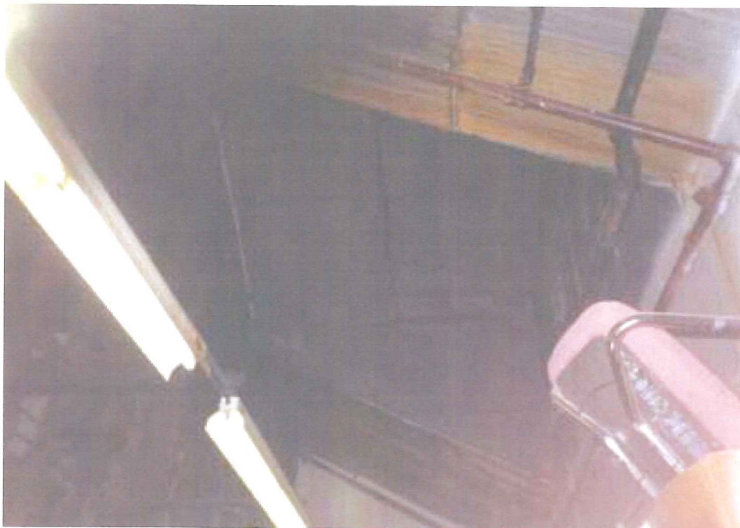
Typical Ceiling and Wall Panels Type 1 Asbestos and Fluorescent Lights
