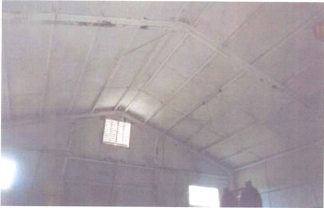
Sprayed On Asbestos Type 2 Steel Structure
