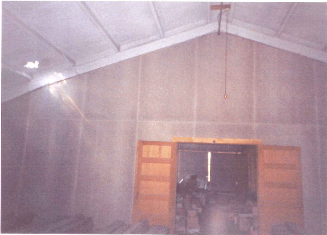
Interior 2 nd Floor - Asbestos Type 1 and Type 2
