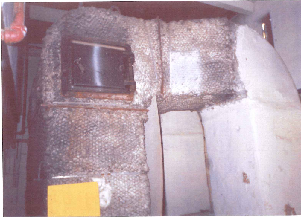
Asbestos Type 2 Pipe Insulation
