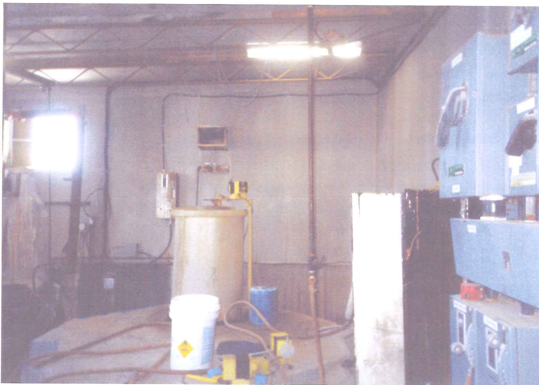
Interior Showing Steel Roof Supports Asbestos Type 1 on Walls & Ceiling and Concrete Pedestal
