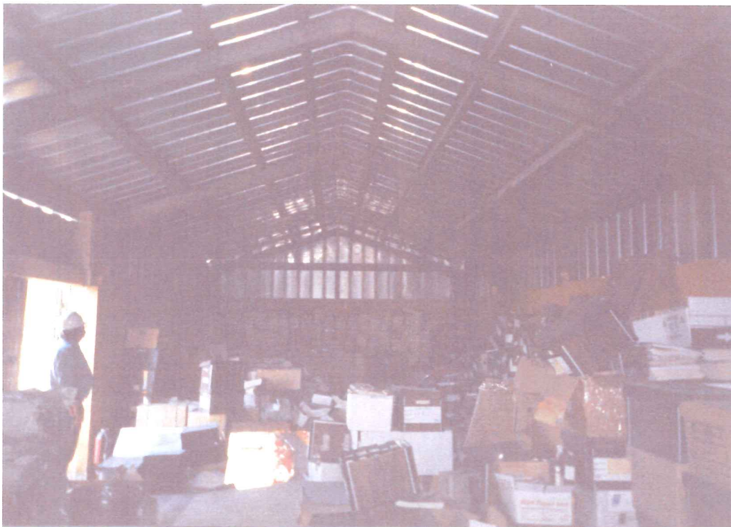
Interior Shows Steel Frame Aluminum Siding & Roofing and Stored Items
