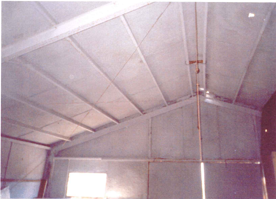
Interior Asbestos Type 2 Steel Frame
