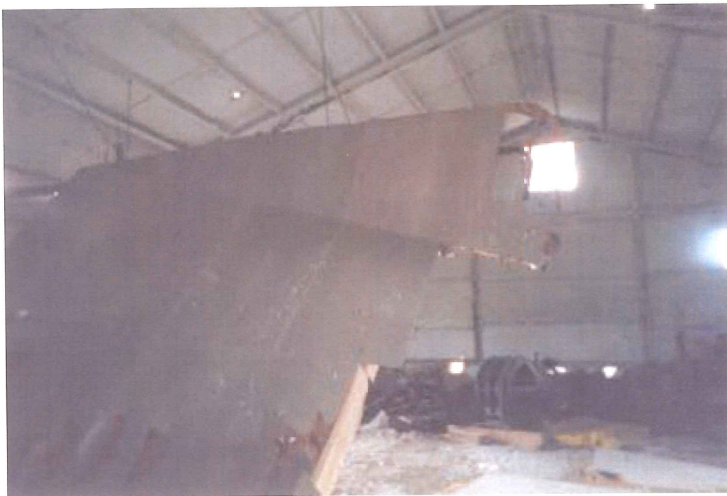
Interior Shows Asbestos Type 1 Wall Panels and Sprayed On Asbestos Type 2 on Super Structure
