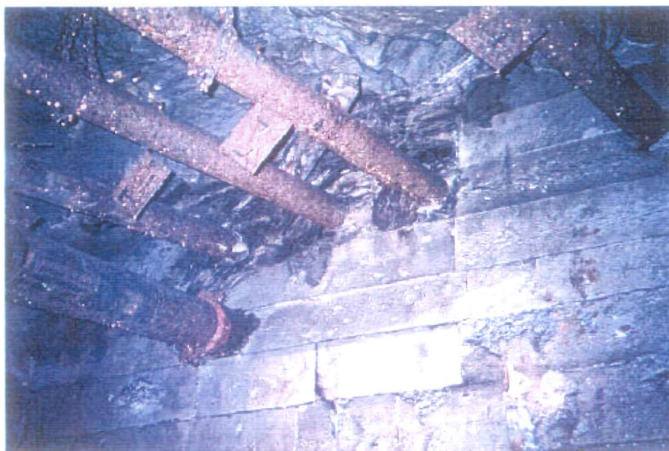
Photo A5-2. Upper bulkhead showing the four 4-inch pipelines used for pneumatic delivery of arsenic trioxide dust and the one 6-inch pipeline for return air.
