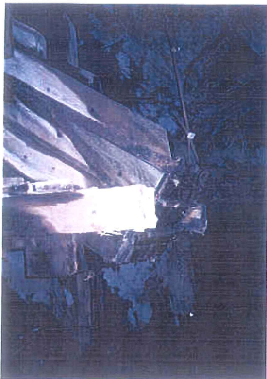
Photo A5-16. Bulkhead #50 in the AR1 area, leading to the C212 shrinkage stope (storage cavern). This bulkhead is the "sandfill type" and on the right there is evidence of leakage.
