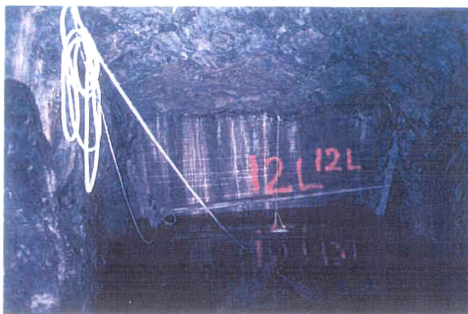
Photo A5-4. The lower bulkhead of the #12 storage cavern, partially flooded.
