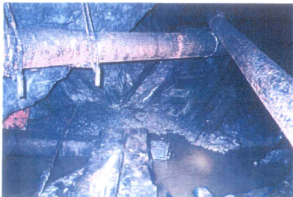
Photo A5-9. The floor of the ADD on the south-east of the main access drift. In this area above caverns B230/33/34/35/36 the conditions are not frozen.
