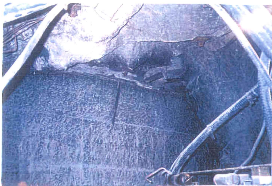
Photo A5-3. The lower concrete bulkhead of the #11 storage cavern.
