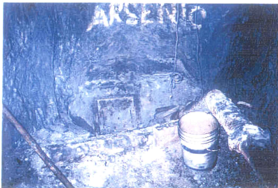
Photo A5-11. The inspection hatch into the storage cavern B208 in the floor of the northern end of the ADD. The floor is covered with frost.
