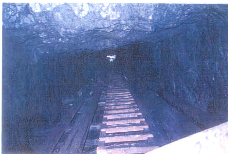
Photo A5-10. Raise and ladder-way to surface at the south end of the ADD.
