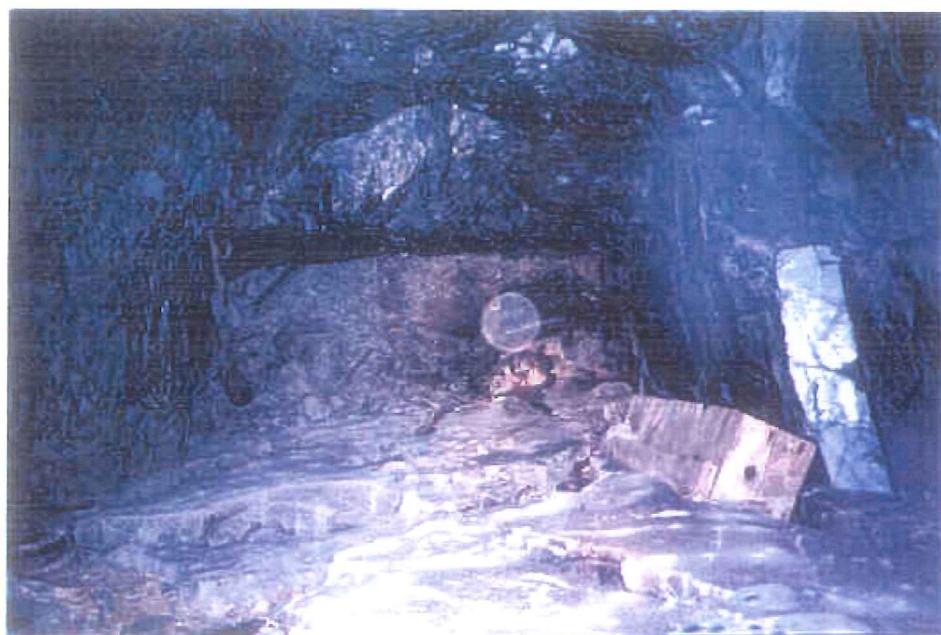
Photo A5-14. The north-west bulkhead at the end of the ADD, leading to the B208 storage cavern. The floor is covered in 4-6 inches of ice.
