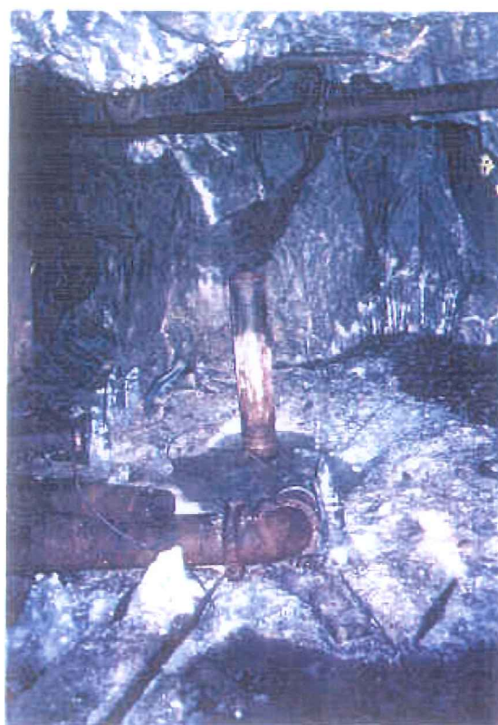
Photo A5-12. The pipelines in the floor of the ADD supplying the B208 cavern with arsenic dust. ice stalagmites and frost on the floor (late September).
