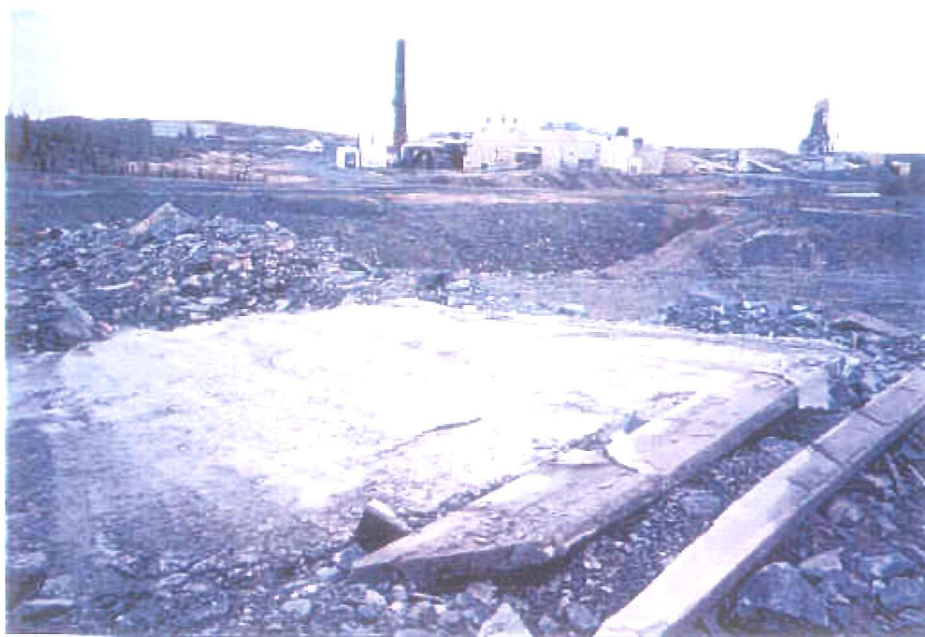
Photo A2-17. Close-up of the capped raise north of B1 Pit.
