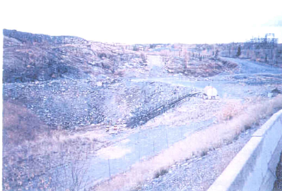
Photo A4-7. C1 Pit, north end, looking north-west. Shows the ladder-way that is part of the emergency escape-way.
