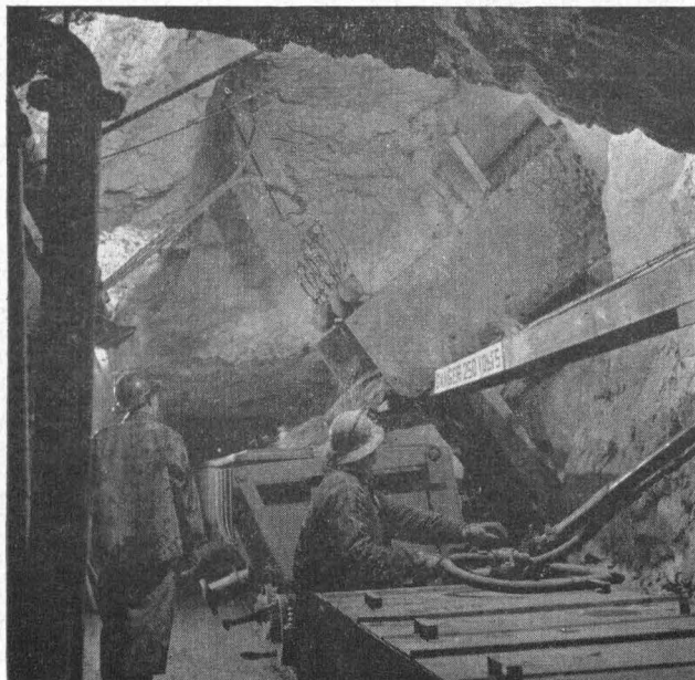
Loading from a steel and concrete chute on the 750 main haulage level.
